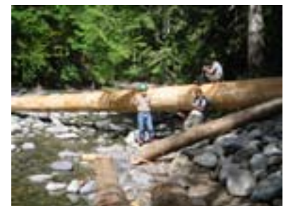
Canyon Creek Footbridge
